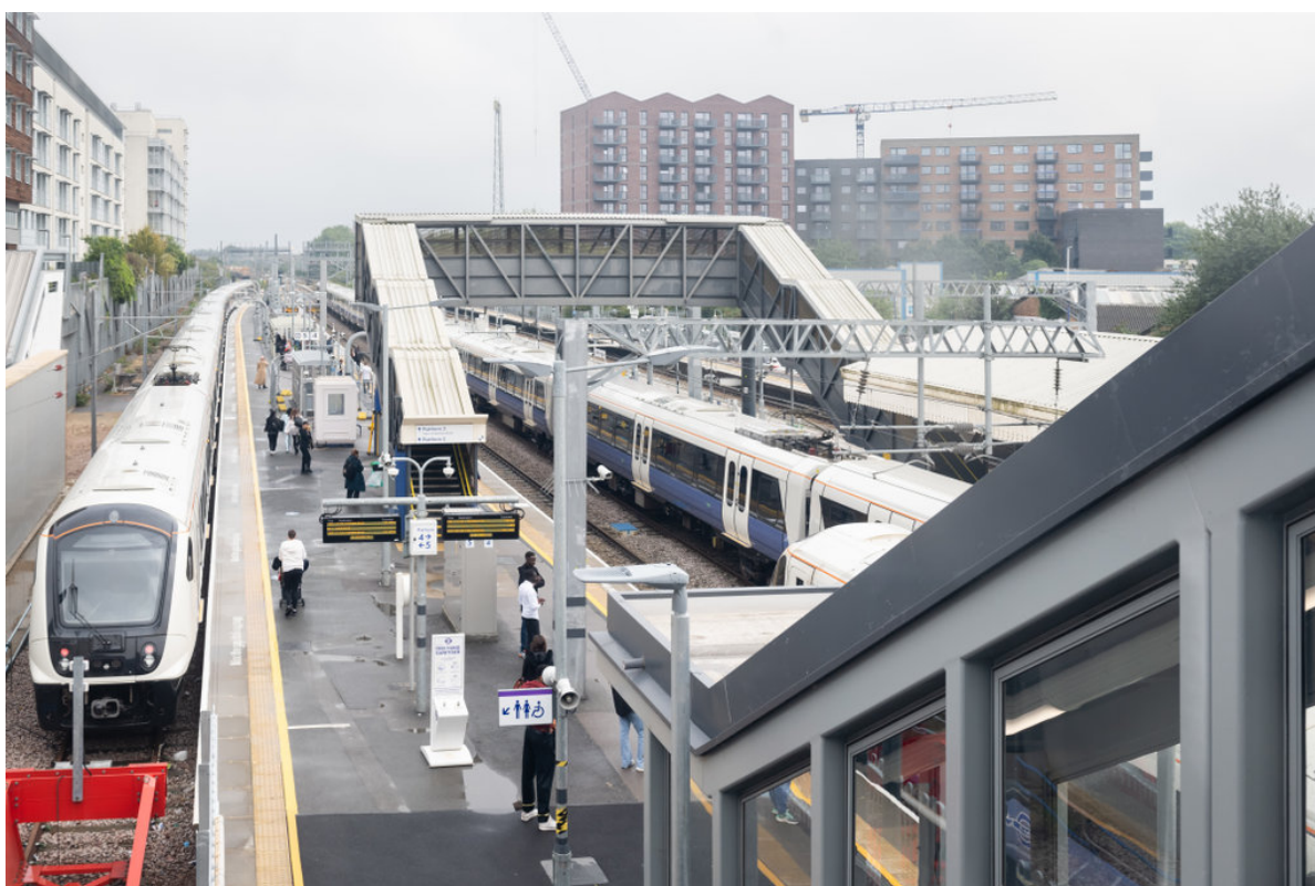
Figure 39. Hayes & Harlington station supporting local development. Source: TfL
