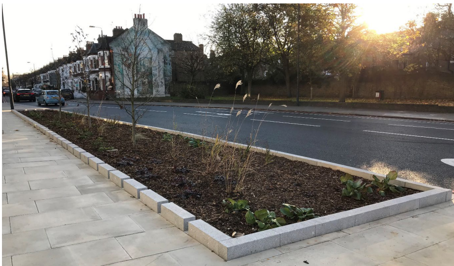
Figure 26. Rain Garden at Elspeth Road, Wandsworth. Photo credit: John Birch, TfL.
