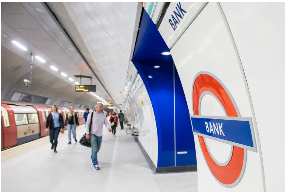
Figure 29. New platform at Bank station after reopening. Source: TfL.
